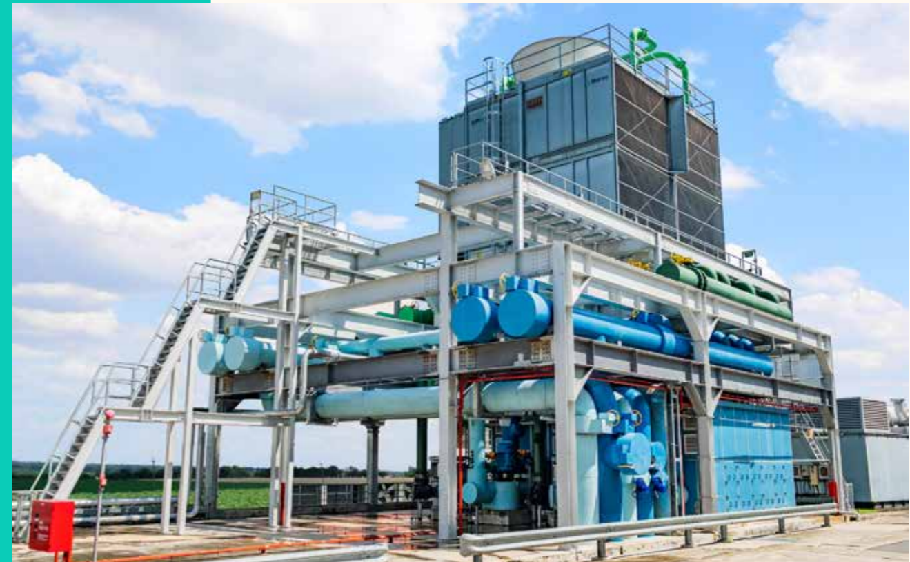
Chillers at PDG's SG1 in Singapore
